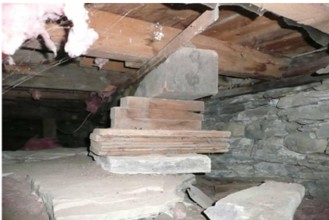
House foundation from 10 years ago
