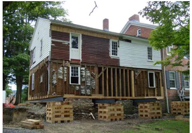
Working on the restoration
