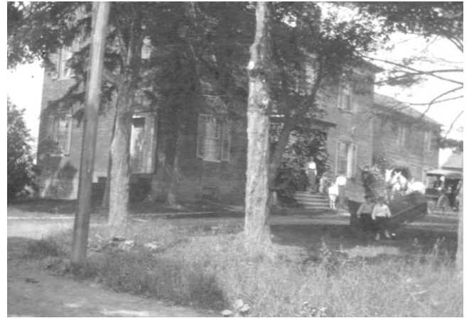
Southworth Homestead ca 1900 showing the west (and south) stair.
