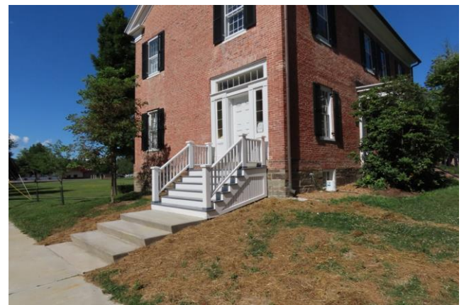
West Stair and New Shutters
