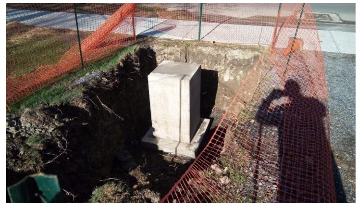
Setting the bases for the reconstructed entrance columns
