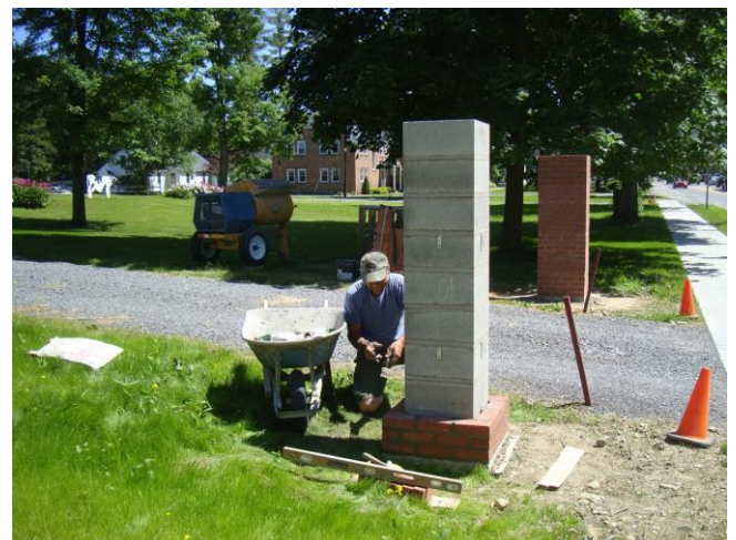
Mason at work on the Southworth Homestead entrance piers.
